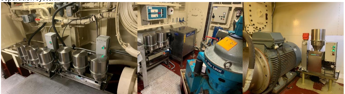
Two pcs. WP1-P2-750 Lubricatin fine filter systems for the two MaK engines
